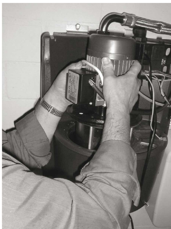
Abb. 29: Pumpenaggregat herausheben
